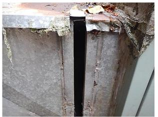
Missing air filter at the package unit
