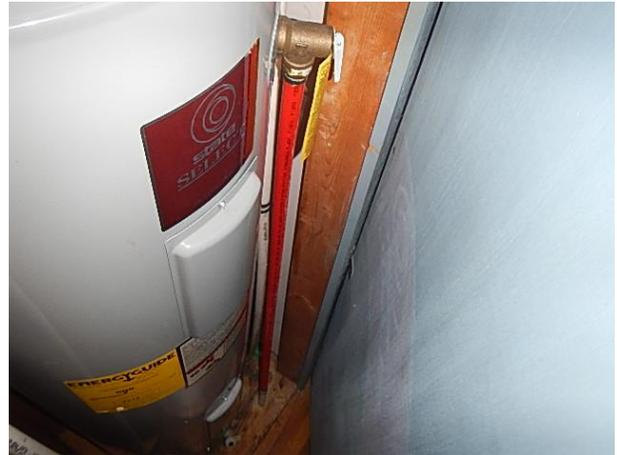
TPR discharge pipe discharges into the crawl space
