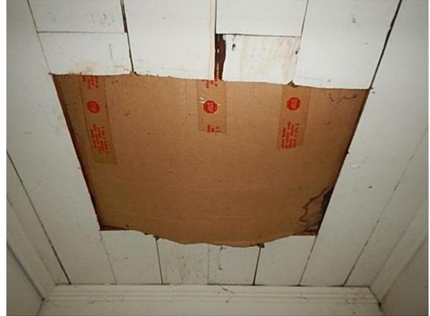
Recommend replacing the cardboard with plywood
