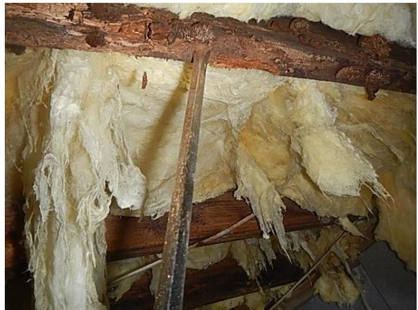
Wood decay at several floor joists
