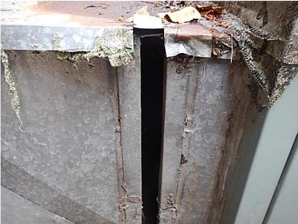
Missing air filter at the package unit
